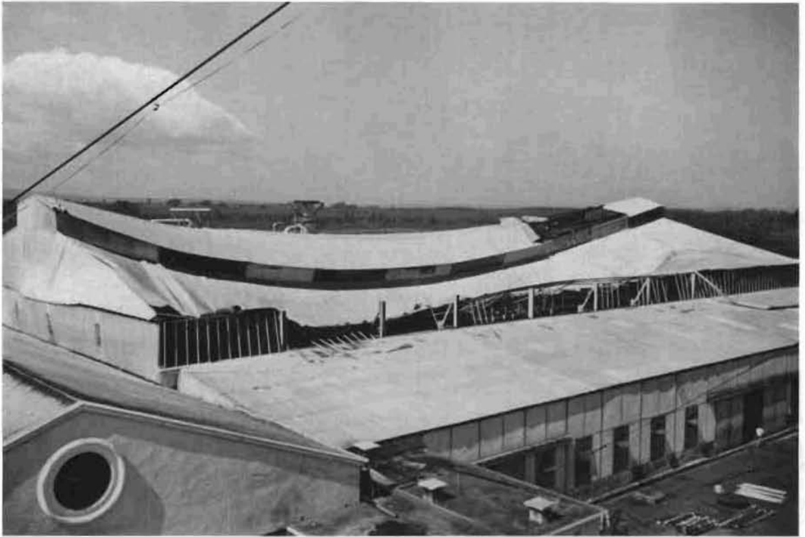
Fig. 15. Union St. Aubin factory after cyclone 'Carol' (above) and Solitude factory after cyclone 'Alix' (below).
