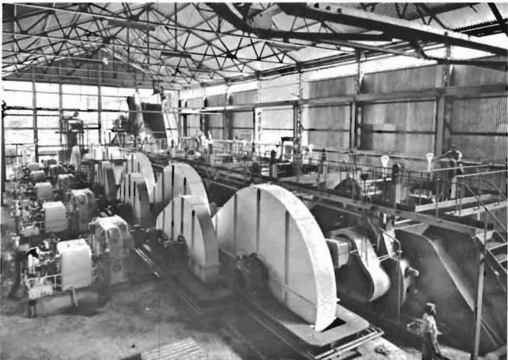
Fig. 40. Turbine driven crushing plant installed in 1958 at Beau Champ factory. ( Phot. P. Halbwachs ).
