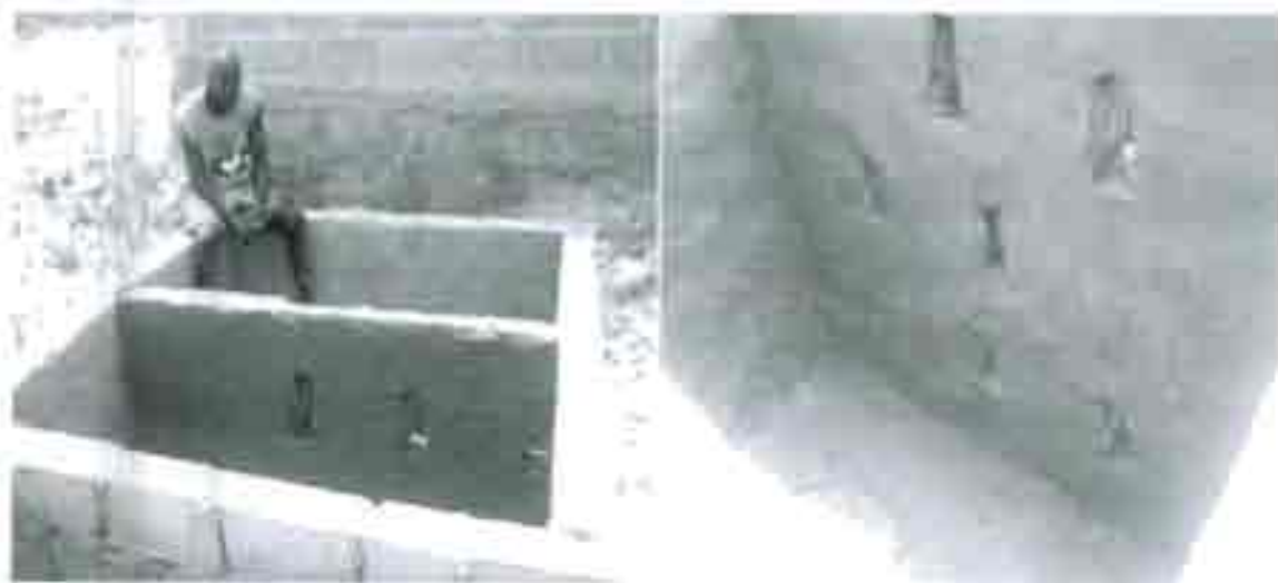
Figure 5: Fosse septique en construction
